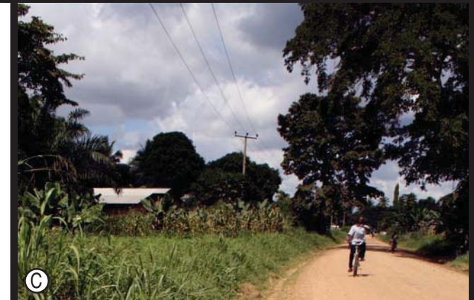
Electric poles are within road right-of-ways but land below them is still traditionally used for agriculture and other uses.
