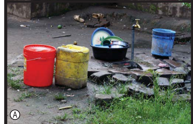
Stand Pipes are a primary water source for many villagers. The pipes bring water from springs and streams into the village.
